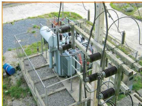
GENERATOR TRANSFORMER 9.5MW BIO MASS BASED POWER PLANT AT KRABI THAILAND
