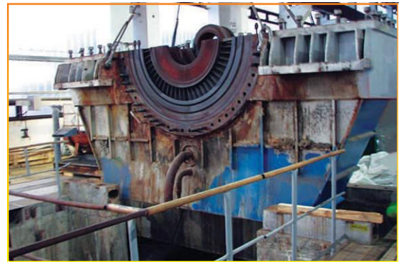
30 MW TG - DISMANTLING UNDER PROGRESS IN BERLIN
