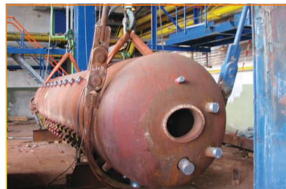
STEAM DRUM ERECTION UNDER PROGRESS 150TPH OIL AND GAS FIRED BOILER IN BERLIN
