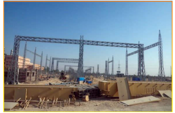
220 KV SWITCHYARD UNDER ERECTION FOR 160MW COMBINED CYCLE POWER PLANT PROJECT AT RAMGARH IN RAJASTHAN
