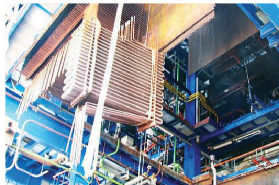
ECONIMIZER ASSEMBLY DISMANTLING UNDER PROGRESS - 150 TPH OIL & GAS FIRED BOILER, BERLIN
