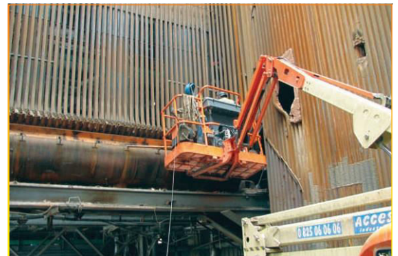
DISMANTLING WORK UNDER PROGRESS 1*15 MW POWER PLANT BOILER IN SWEDEN
