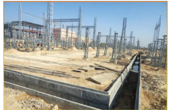
CABLE TRENCH-160 MW COMBINED CYCLE POWER PLANT PROJECT AT RAMGARH IN RAJASTHAN
